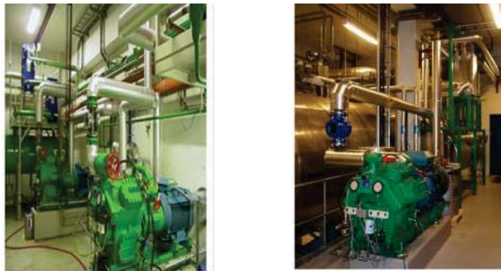
Figure 3-11: Pictures of two “hybrid” heat pumps by “Hybrid Energy AS” left: 300 kW, right: 650 kW heating capacity [Nordtvedt, 2009]
