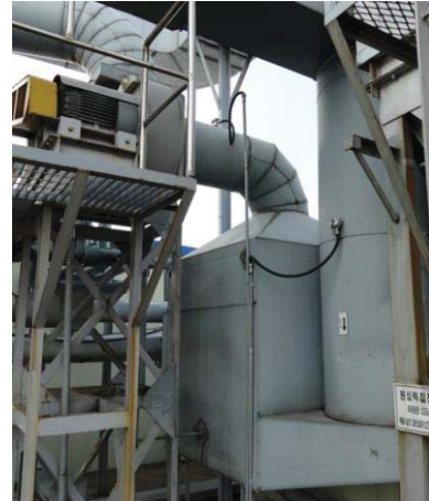
Figure 9-4: Schematic diagram of water-fluidized bed heat recovery system and its installation scene
